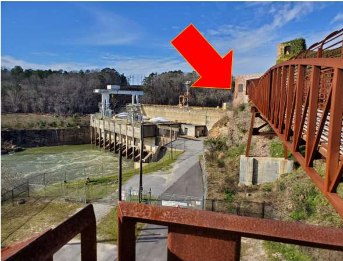
Photo of the North Highlands Dam with the approximate location of Lovers Leap noted by the arrow. A pedestrian bridge leading to the mill ruins is on the far right.
