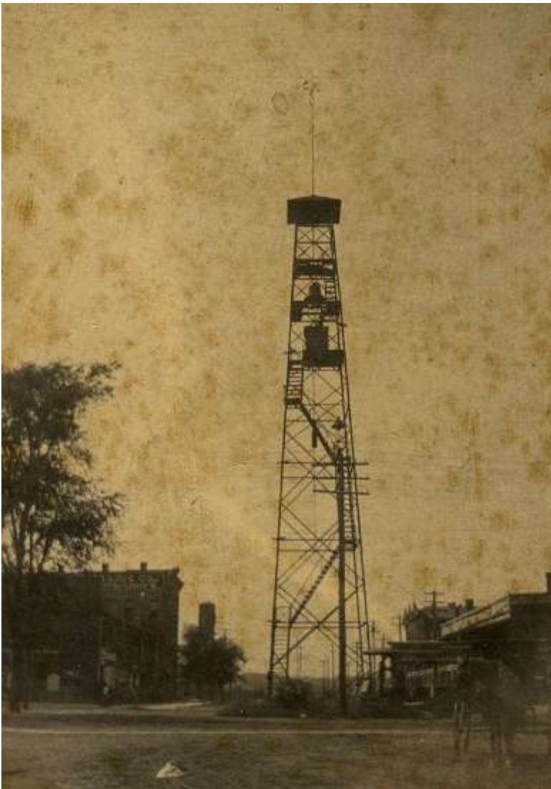
Photo of the Fire Alarm Bell Tower, courtesy of the Columbus Museum, https://columbusmuseum.pastperfectonline.com/webobject/213870CD-42E3-418B-92DA-228341059490
