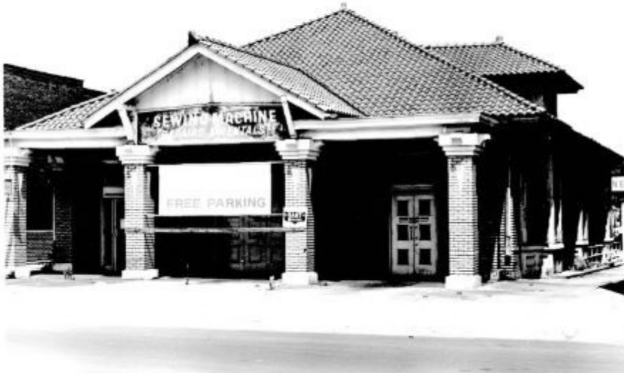
Fire House #1 as it appeared in 1980 (National Register nomination).
